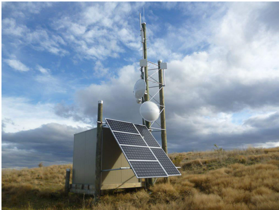
Figure 2.5.4. Wireless access point antenna installed on a hillside overlooking a town.
