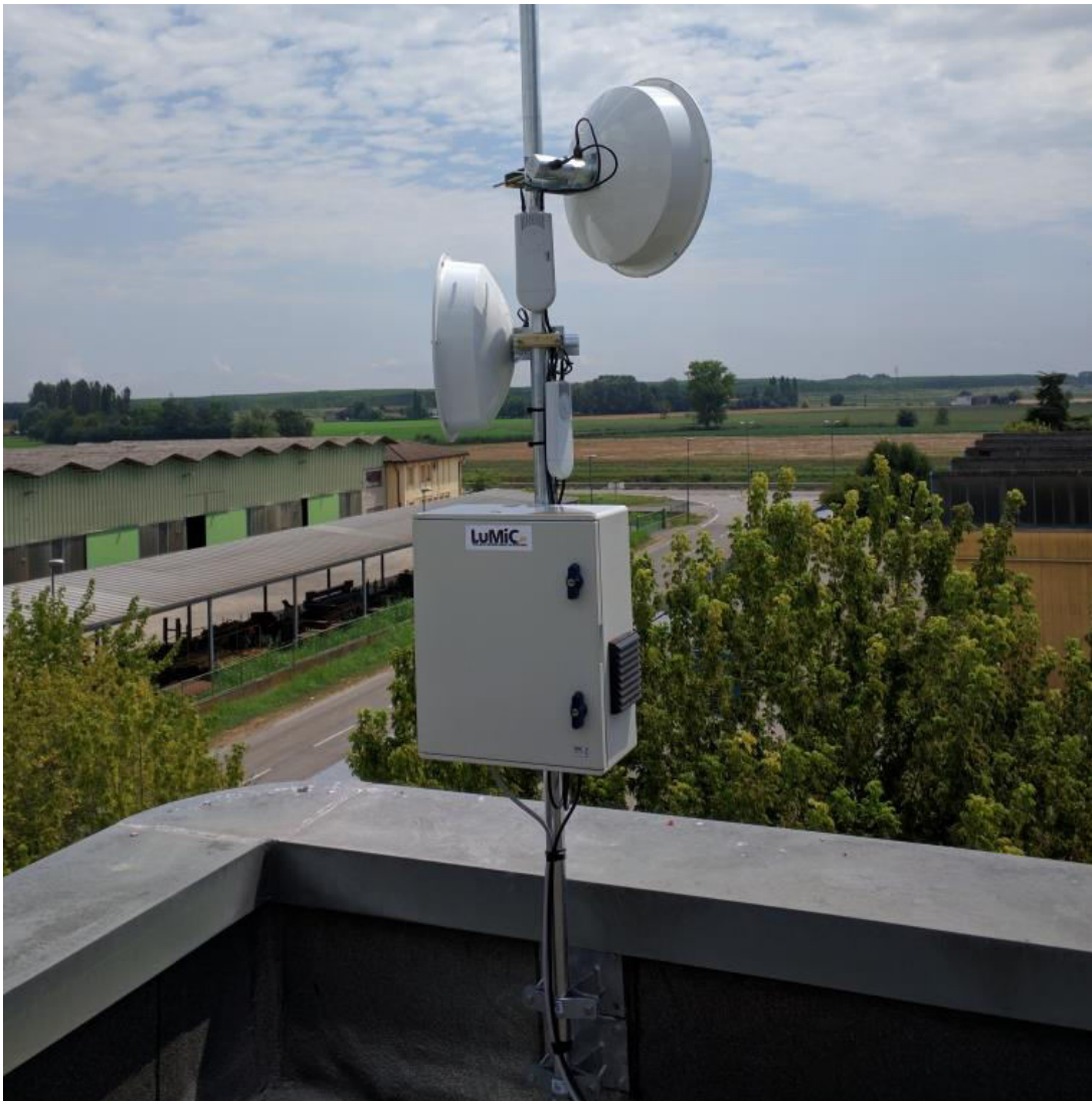
Figure 2.5.8. Relay/repeater antenna to extend the distance between the PtMP tower and the network operations center and for non-line-of-sight connections.
