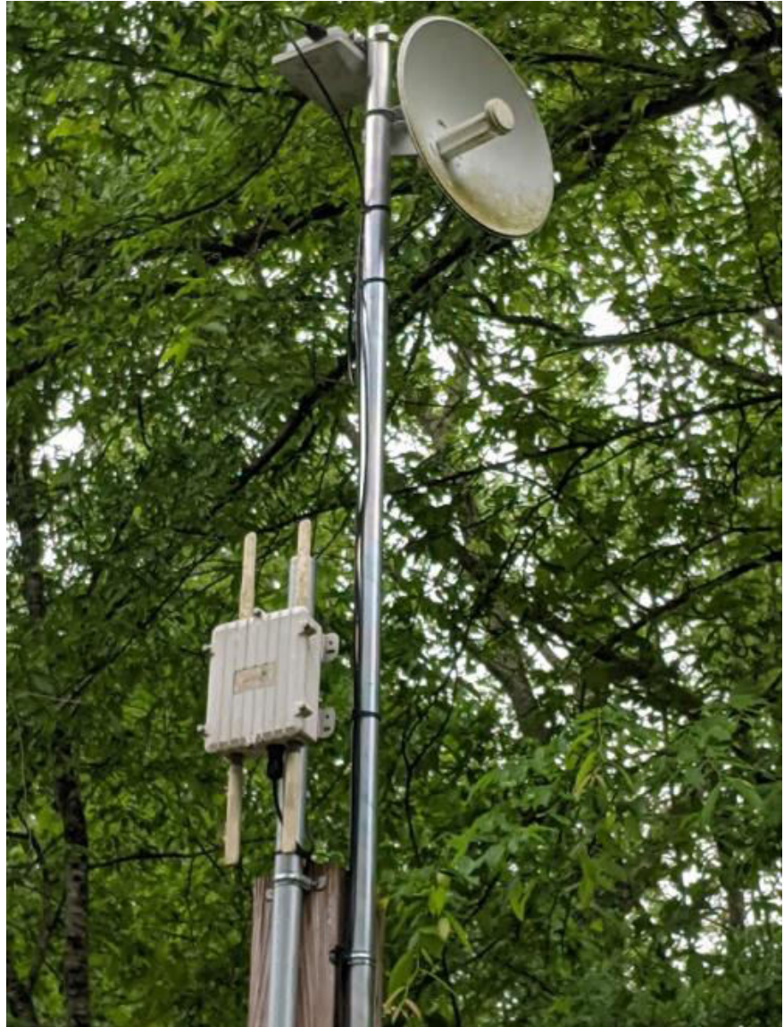
Figure 2.6.1. A mobile broadband campground Hotspot installation with a PtMP wireless access point and a PtP backhaul antenna provides Internet for visitors and an on-demand charge is made for the service.
