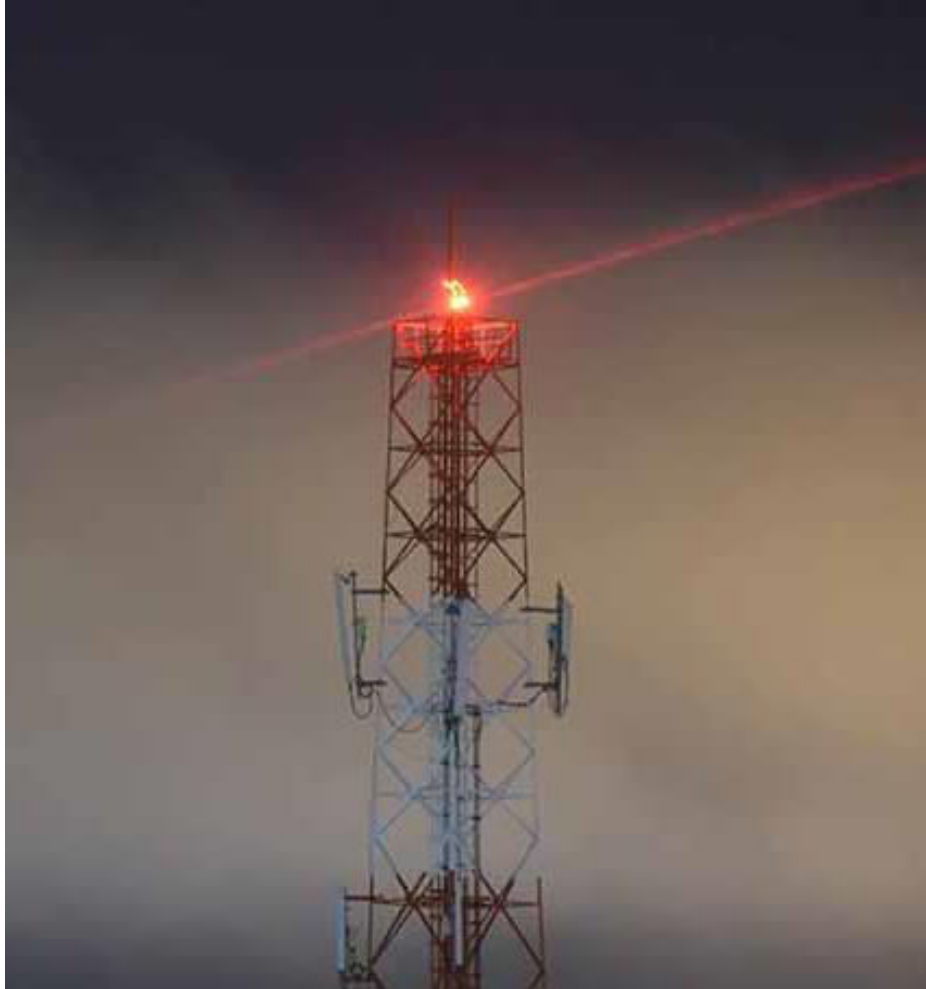
Figure 2.14.4. Antenna tower warning light for aviation.
