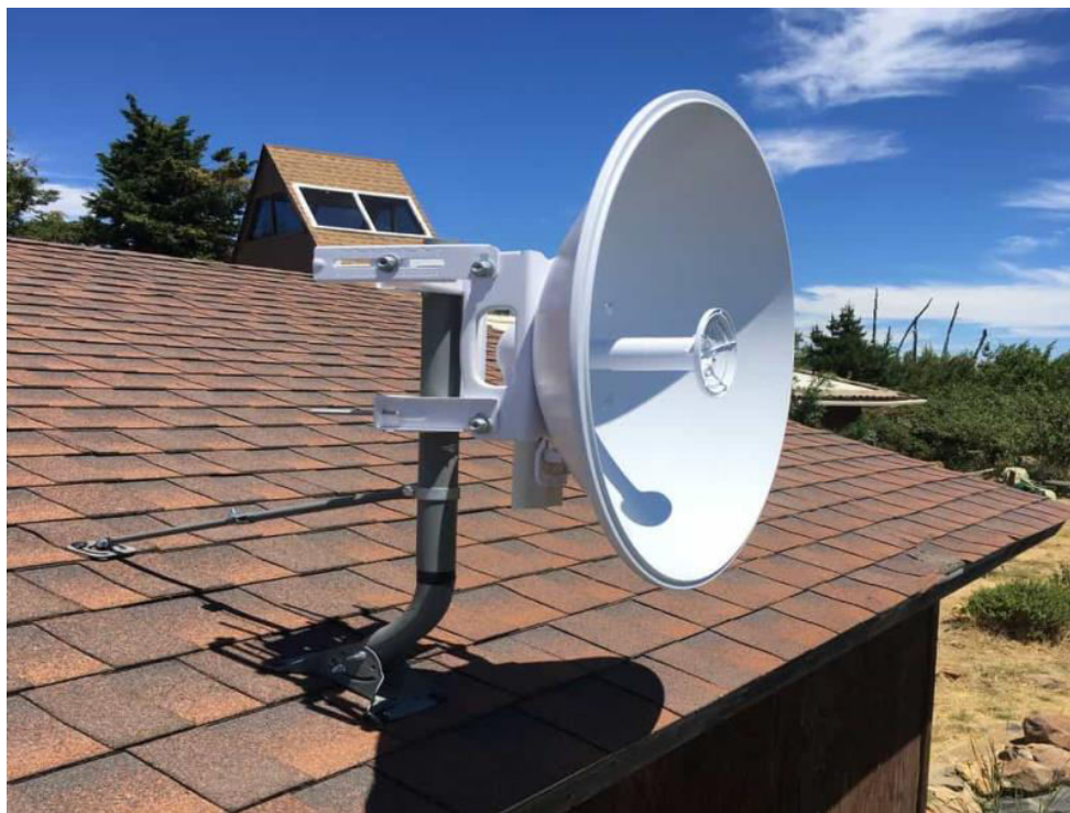
Figure 2.9.6. CPE parabolic antenna installed on the roof of the subscriber's building.
