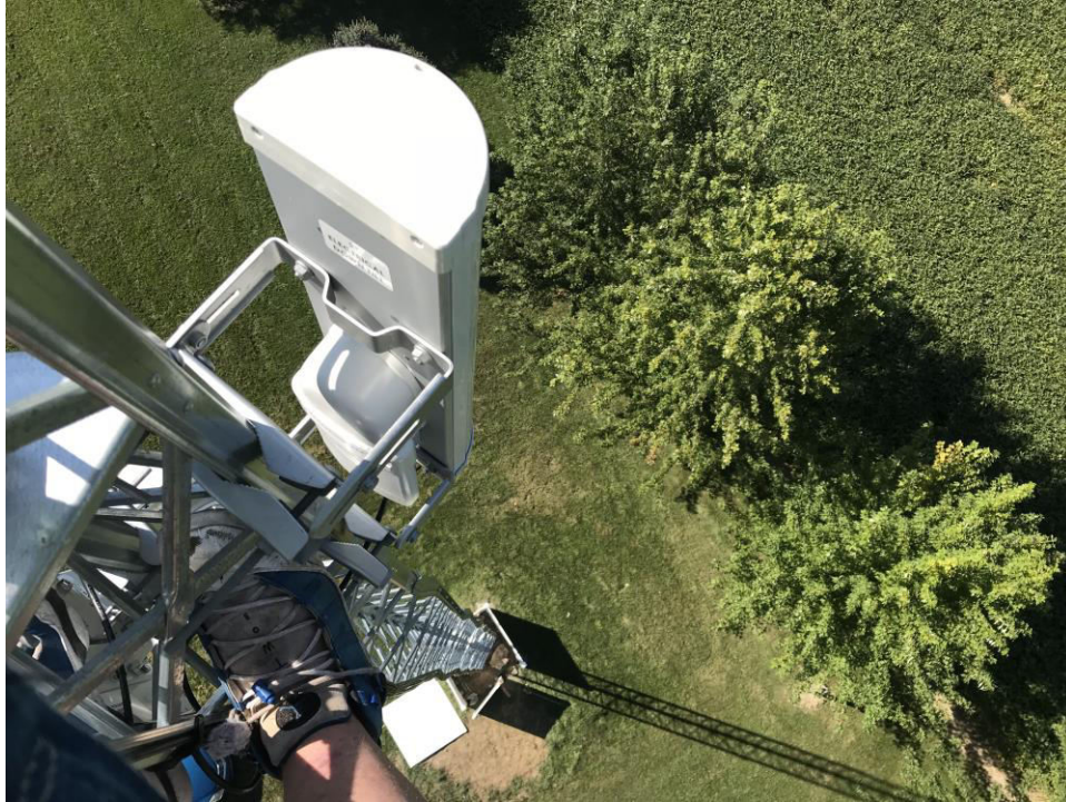
Figure 2.5.3. Wireless access point antenna installed on an antenna tower.
