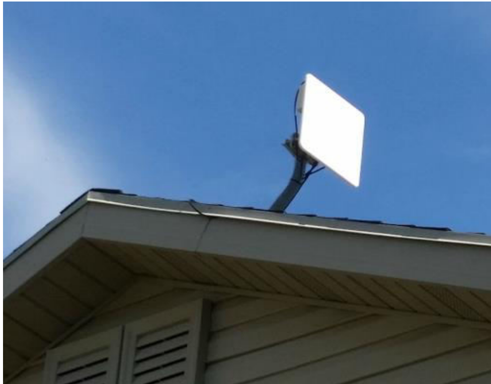
Figure 2.9.4 CPE panel antenna installed on the roof of a subscriber building.
