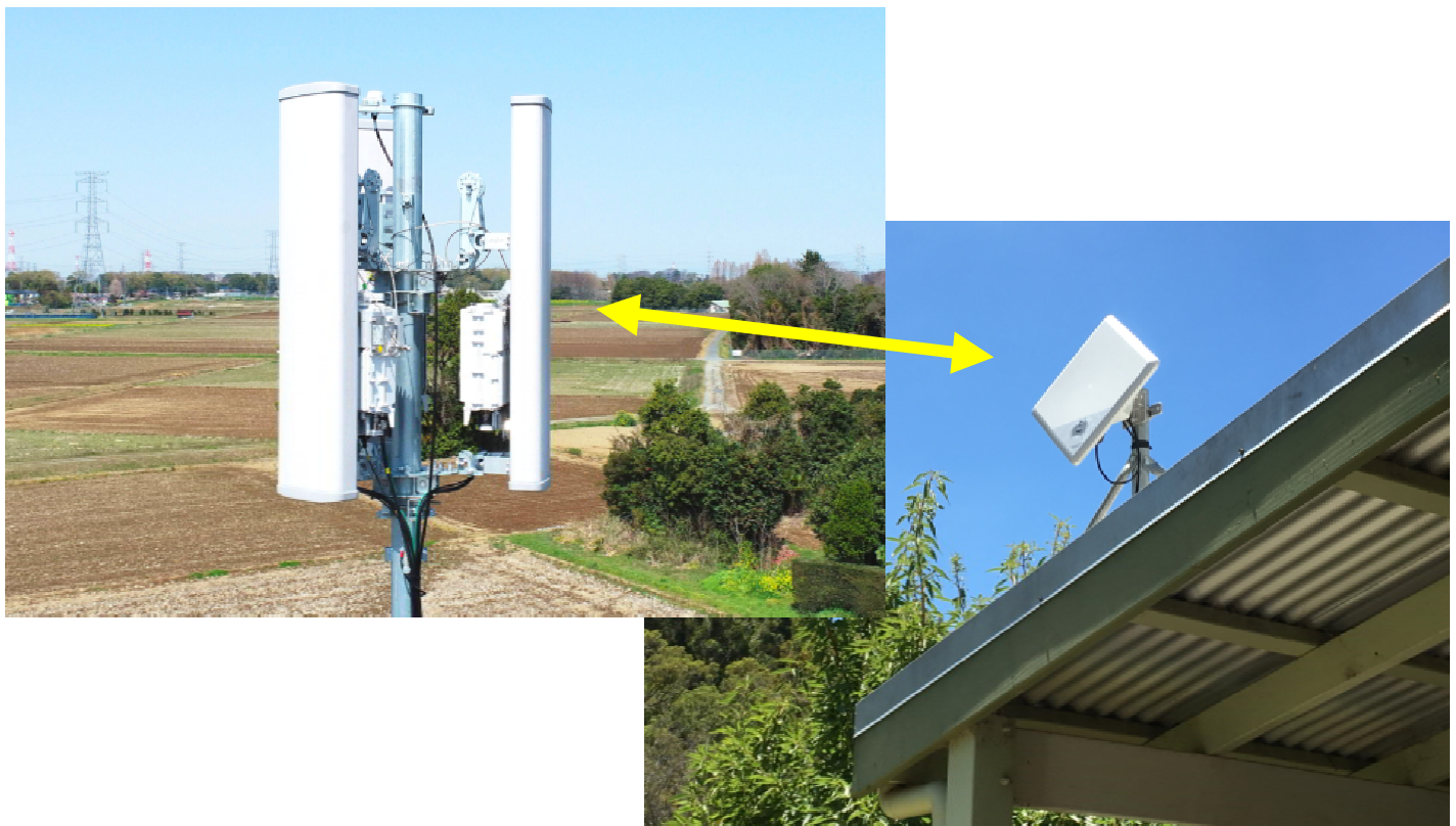
Figure 2.5.9. CPE antenna installed on the roof of a subscriber building.
