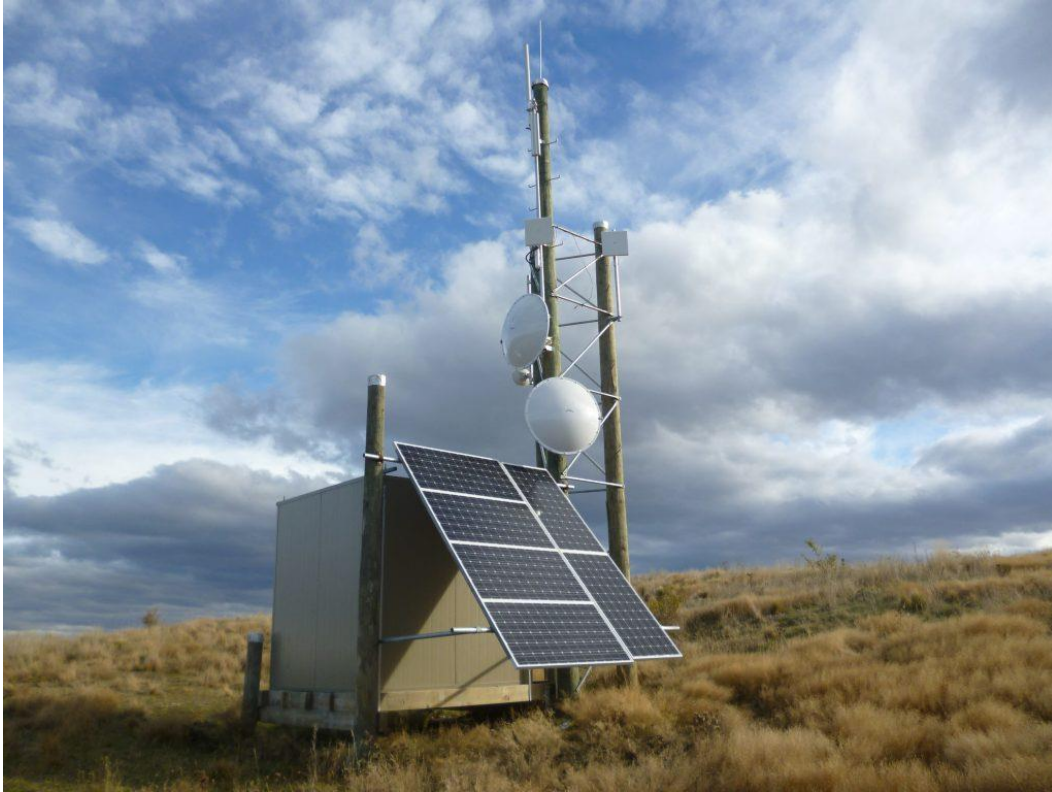
Figure 16: Wireless access point antenna installed on a hillside overlooking a town.
