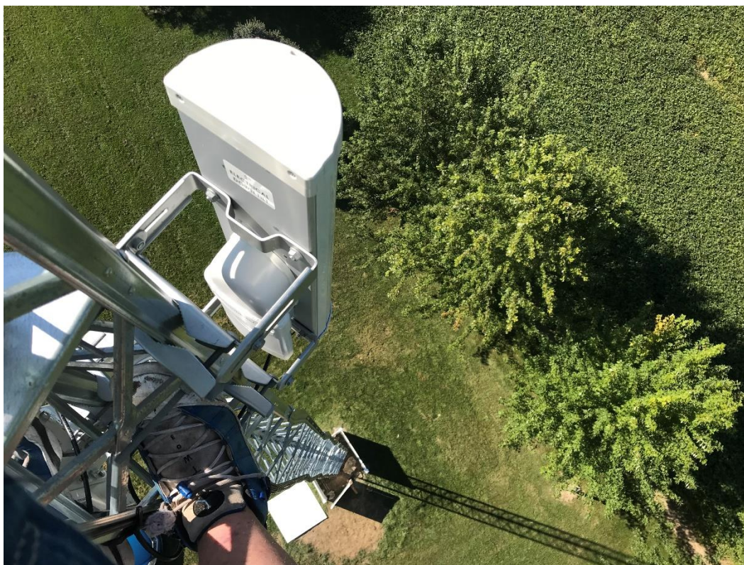
Figure 15: Wireless access point antenna installed on an antenna tower.
