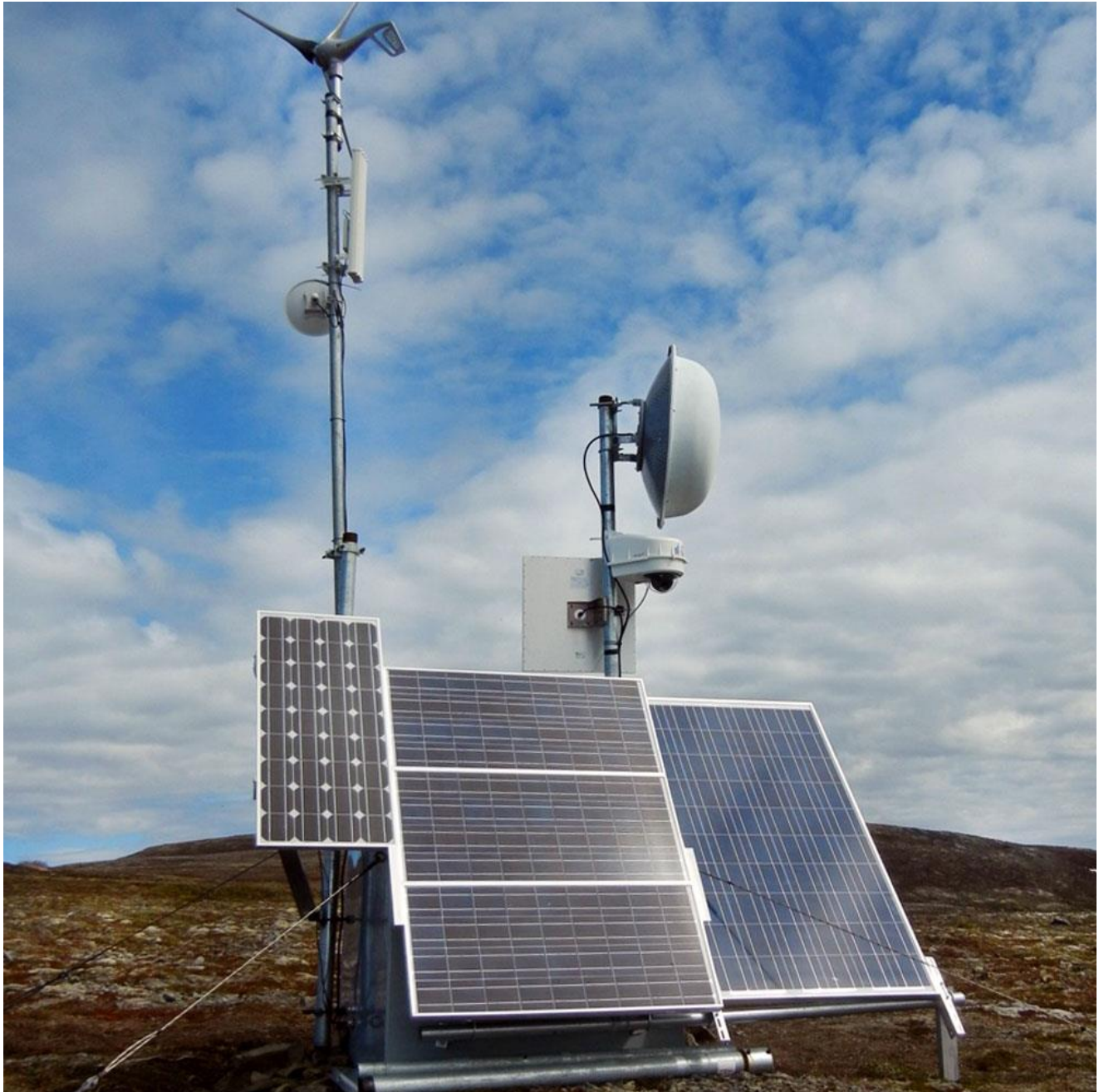
Figure 26: Hilltop PtMP antenna installation with backhaul antennas and solar panel power supply.
