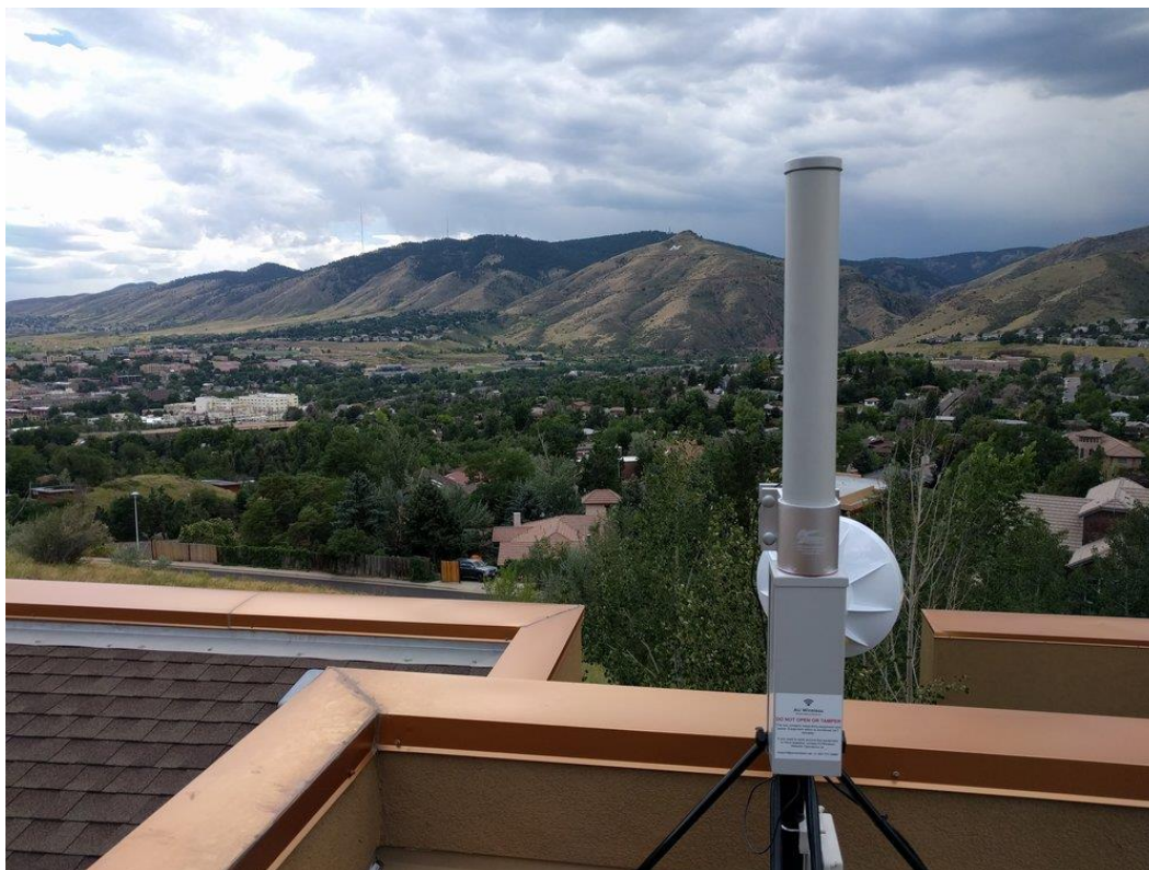
Figure 14: Wireless access point antenna installed on a building roof.
