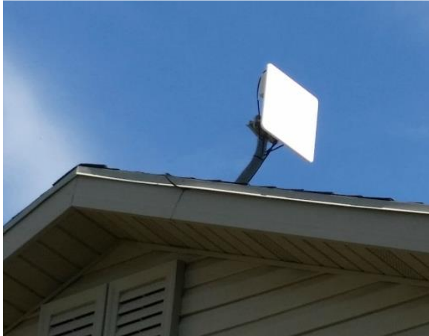
Figure 12: CPE antenna installed on the roof of a subscriber building.
